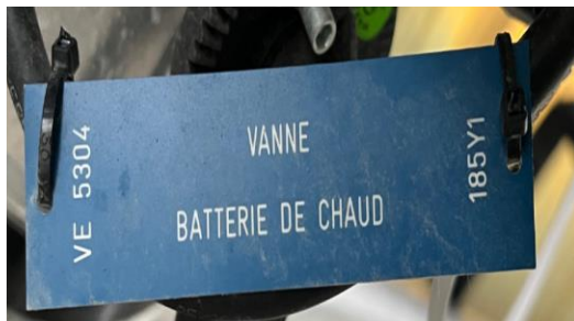
Figure 115 : Installation de ventilation
