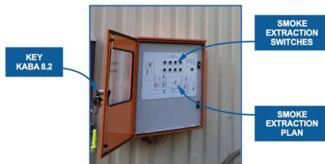
Ventilation box example
